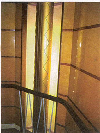
Custom vertical basket indirect luminaire for the Ocean Liner MS Regal Empress stair tower landing built by Alexander Stephens and Sons of Glasgow. Photo by Peter Knego
